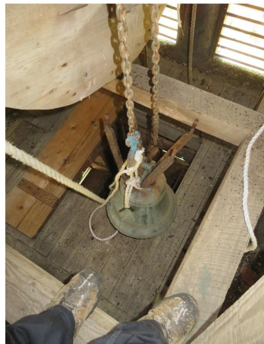
Figure 3. The inscribed bell removed and lowered before wrapping. The bell, estimated at 70-80kg, was considerably lighter than the shield bell, weighing in at approximately 100kg.
