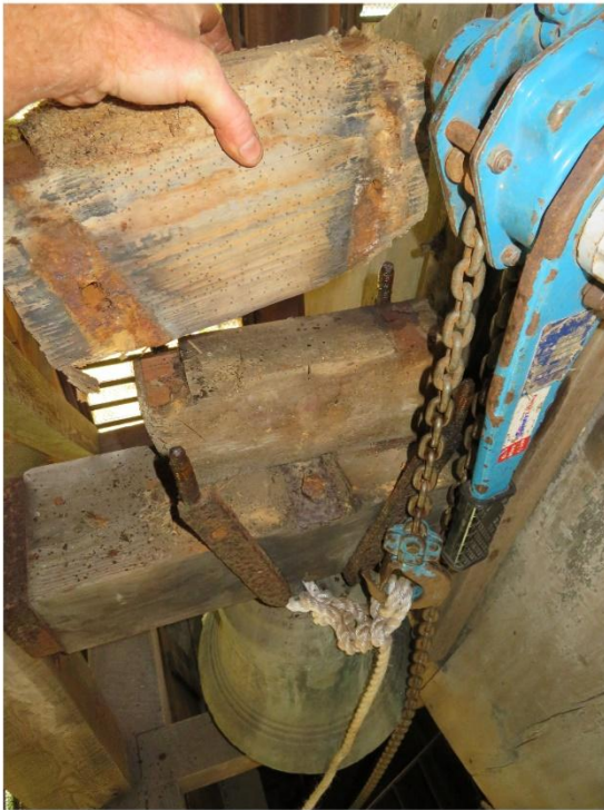
Figure 2. The badly degraded head stock and strapping is carefully removed before the shield bell is secured, wrapped and lowered to the ground floor.
